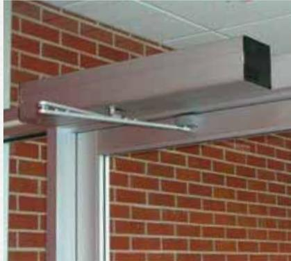
Single—side load lintel mounted header
