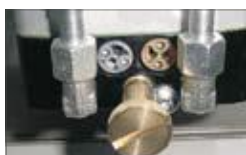
By pass valves
